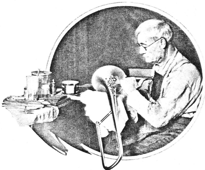
Hand burnishing a mirror surface; the last step in making an OLDS trombone.
